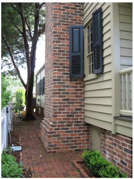
The elevation of this dwelling included rebuilding the base of the chimney with brick and mortar to match the original (Beaufort, South Carolina).
