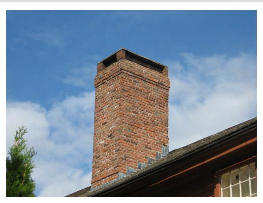
Most chimneys in the Newport Historic District are of brick and are located on the interior rather than on exterior walls. In an elevation project these chimneys should be elevated along with the rest of the house and kept at their original locations (above, 59 Bridge Street and below, 54 Thames Street).
