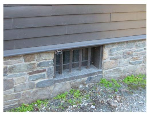
If wet flood proofing is considered, utilize existing openings such as basement windows for the installation of flood vents if the opening is at least one-foot above grade (Above: 39 Washington Street, Below: 11 Third Street).
