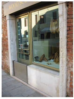
Examples of flood shields to protect entrances. The photo above shows a shield and shield track in deployed position (Venice, Italy).
