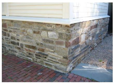
Many Newport houses were built with solid stone foundations. The elevation projects at 74 Bridge Street (above) and 78 Bridge Street (below) added additional stone courses in keeping with the original designs.
