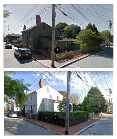
70 Bridge Street in July of 2012 (top) and after elevation in September of 2019 (bottom). Landscaping, staircase configuration, fences, and foundation treatment all contribute to the elevation design.
