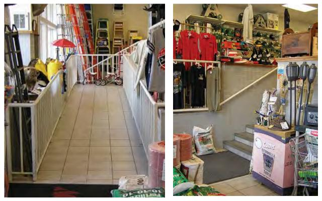
After entering the business, shoppers can either go up the ADA compliant ramp (left) or go up the stairs to the new first floor level (right). The entrance area has been retrofitted with flood resistant materials including a tile floor and tile surfaces on the stairs (Darlington, Wisconsin, photos courtesy of FEMA).
