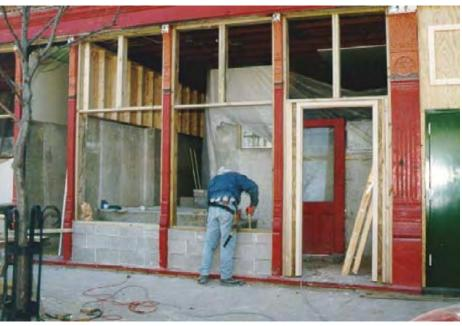
Another strategy for dry proofing commercial buildings is to harden the storefront and raise the interior first floor level. In this approach the frame storefront bulkheads are replaced with concrete and a parged surface (above).
