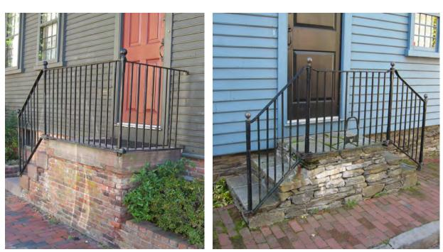
Appropriate stair designs for elevated buildings include the side/linear stair of brick construction at 11 Third Street (left) and the center/linear split wood stair of stone at 6 Bridge Street (right). Both have iron posts and railings in traditional Newport designs.
