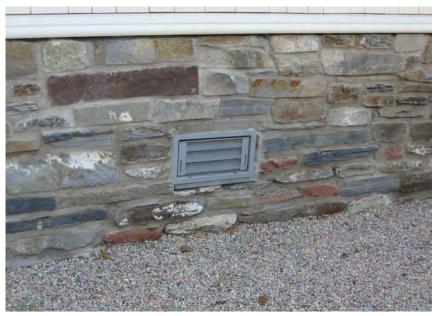
Example of a standard size flood vent and appropriate location onefoot above grade at 74 Bridge Street.
