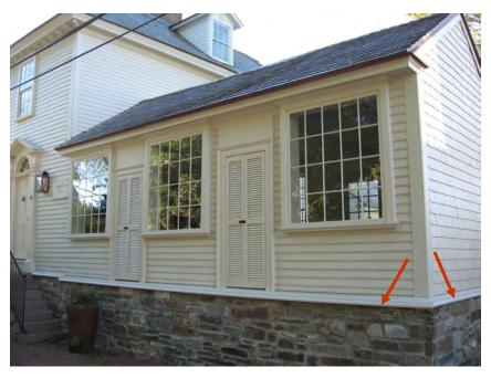
*The elevation of 74 Bridge Street included the addition of a wide water table between the foundation and wood siding.*
