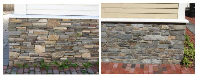
The rebuilt foundations at 62 Bridge Street (left) and 31 Walnut Street (right) reused existing stone and were designed to complement the original designs.
