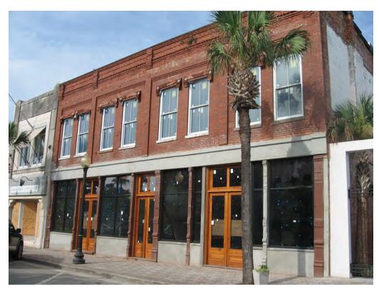
The rehabilitation of this historic commercial building included the hardening of the bulkheads (the panels beneath the display windows) through the replacement of the wood panels with concrete and a parged surface to withstand flooding (Brunswick, Georgia).
