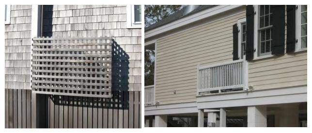
Screening of utilities may include the use of lattice panels (left) or traditional railing designs (right). In both projects the utilities were placed at the rear elevations (left, Nantucket, Massachusetts and right, Mandeville, Louisiana).
