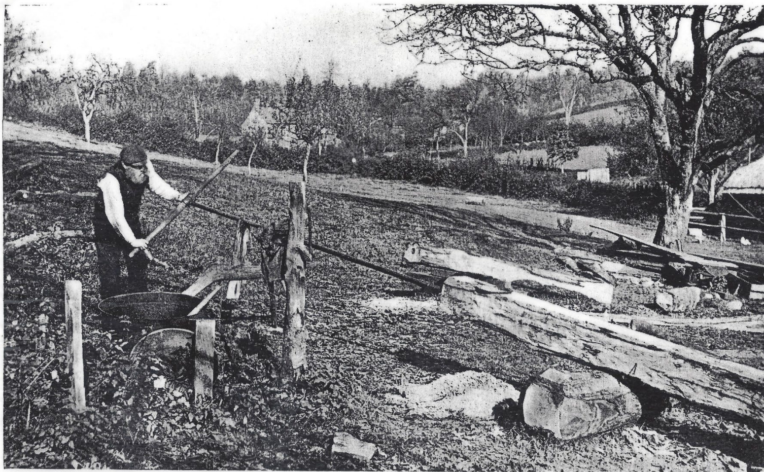
61 Boring elm water-pump pipes by hand, using an auger supported on a rest; Lugwardine, Herefordshire, about 1900
