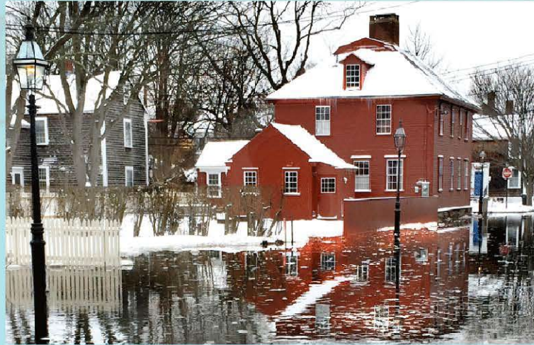
Flooding at 74 Bridge Street, 2016
