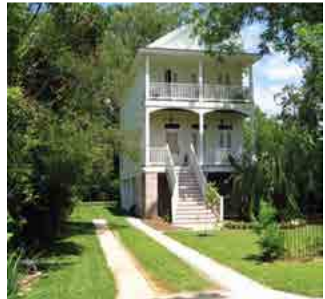
Driveways and parking areas can have significant influence on the appropriate elevation option.
