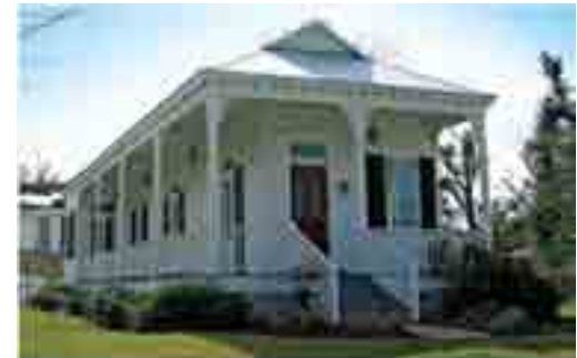
Foundation plans should be scaled to the height of the new base elevation.
