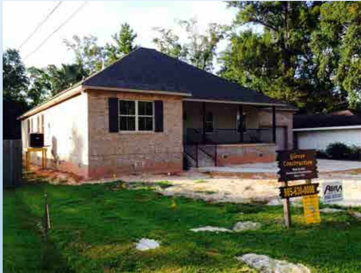
LOW ELEVATION WITH FLOOD VENTED ENCLOSURE
