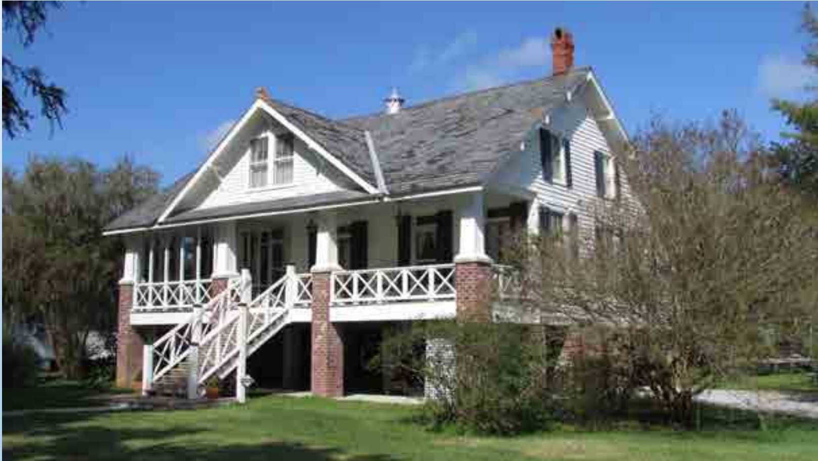
HIGH ELEVATION OPEN FOUNDATION
